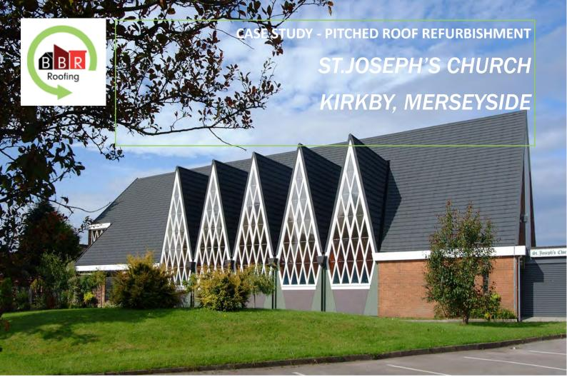
When it became time to renew the old tiled roof of this local parish church, the client opted for a durable and robust roof covering in metal, but with the aesthetic appearance of traditional tiles.
