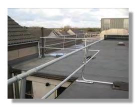
An Index Total waterproofing system incorporating vapour barrier, thermal insulation, underlay and mineral surface cap sheet, all torch-applied was installed to the flat roof areas.
