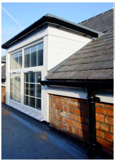
The dormer windows, flat roofed along the internal valley, and barrel roofed on the external elevations, were re-waterproofed with SIKA Decothane and re-clad on the external faces with upvc cladding and fascia boards. The windows were also replaced in upvc frames and double-glazing in a pattern to match the original style of the building.
