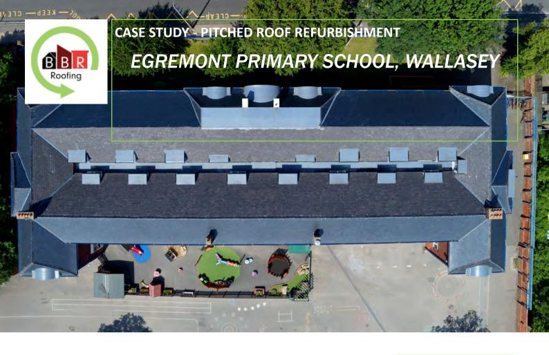
Egremont Primary School on The Wirral required a variety of external waterproofing improvements, which were approved and funded under the Department for Education's Condition Improvement Fund. BBR Roofing were appointed to carry out these works which included roof slating, flat roof waterproofing, external cladding of dormer windows, window replacement, and some internal re-construction works.
