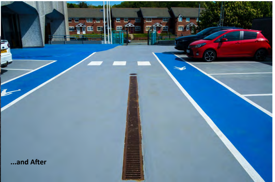
Podium Car park, Before...
