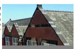
The feature brick gables and coping stones were taken down and rebuilt
