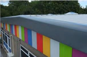
A previously installed pitched roof conversion had blown off the school roof in high winds due to an inadequate fixing system. BBR Roofing were subsequently commissioned to install a new pitched roof over the original flat roof, following a specification produced by consultants AA Projects.
