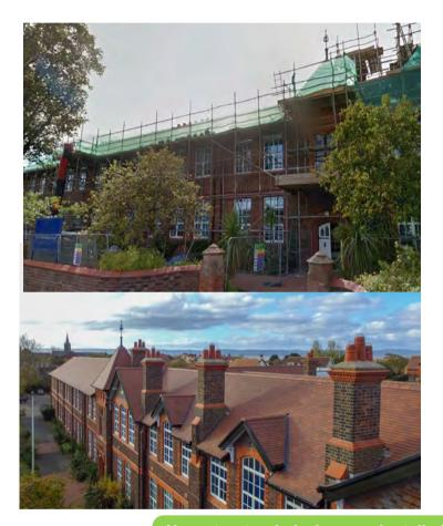
Amongst many other fine details, the cast iron spire over the front main entrance had to be removed, renovated and re-installed.
