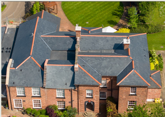
Grade 2 listed Boughton Hall (above)
